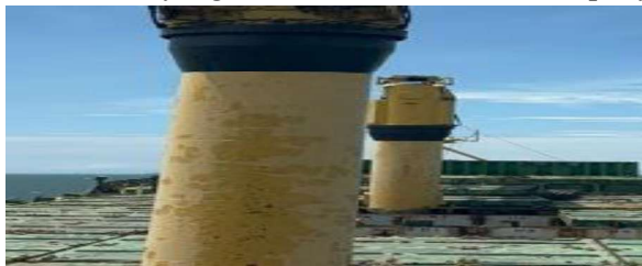
Gambar 2. 11 Tiang Crane/ base structure
