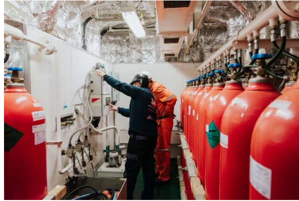
Gambar 2.10 : Fixed fire suppression systems
