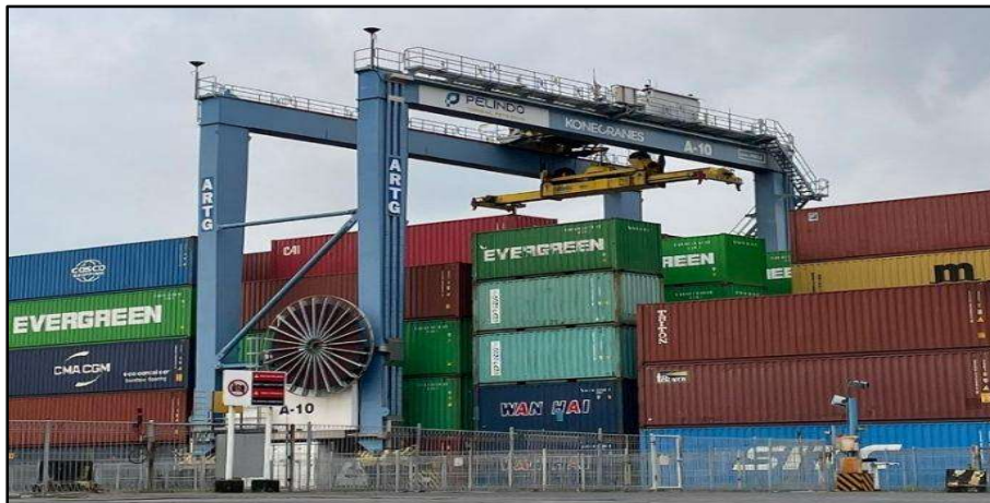
Gambar 2. 2 Automatic Rubber Tyred Gantry ( ARTG )
