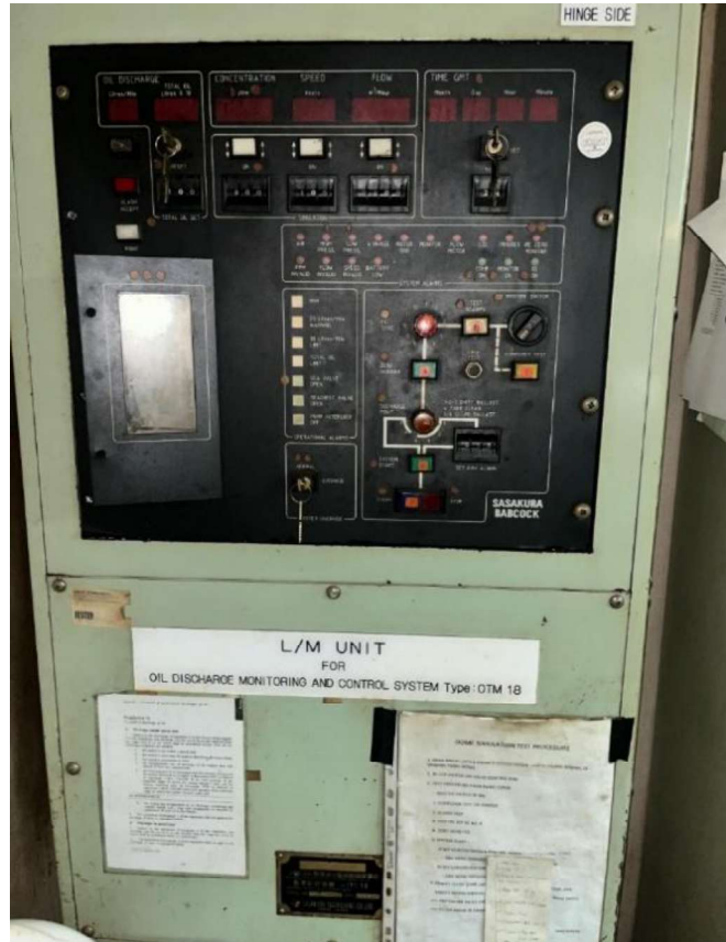
Gambar 2.2 ODM ( Oil Discharge Monitoring )
