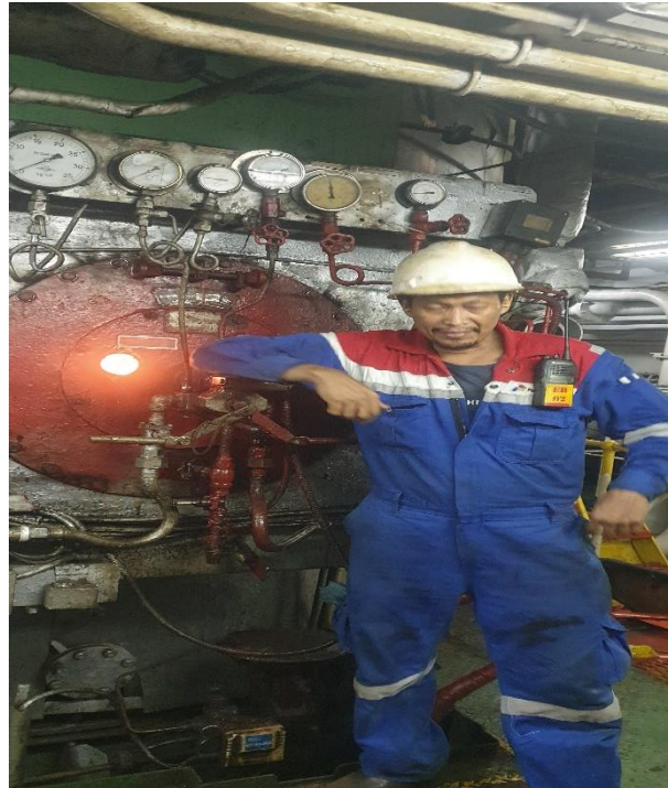
Gambar 2.6 Burner Boiler
