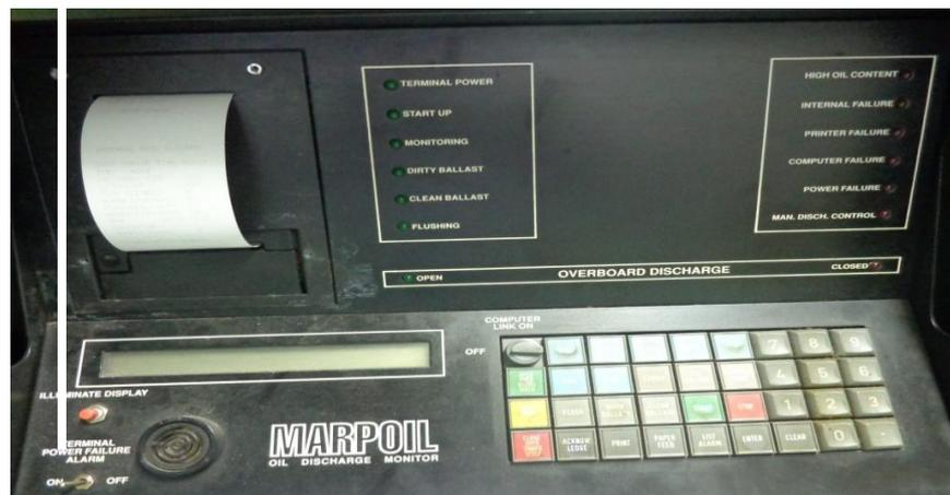
Gambar 2.5 Oil Discharge Monitoring
