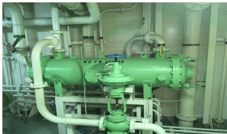
Gambar 2. 4 Fresh Water Cooler
