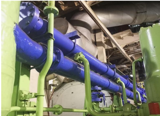
Gambar 2. 5 Fresh Water Cooling Pump
