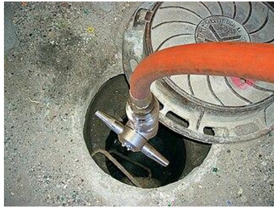
Gambar 2. 5 Proses pengoperasian butterworth
