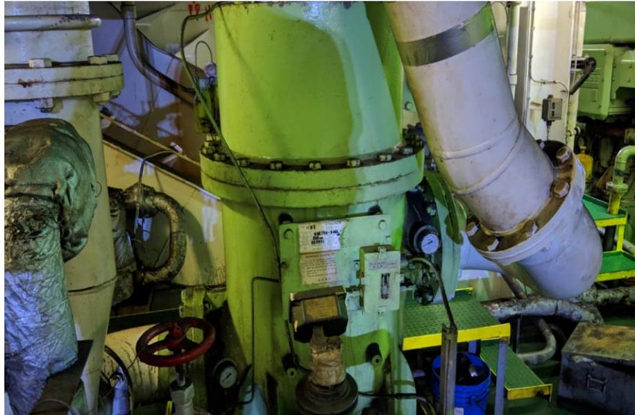
Gambar 2.4 *Filter Lubricating Oil*
