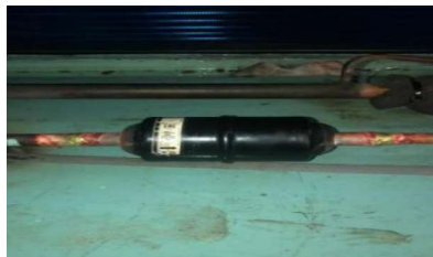
Gambar 2. 7 Filter Dryer Sumber: (Shevchenko et al., 2023)
