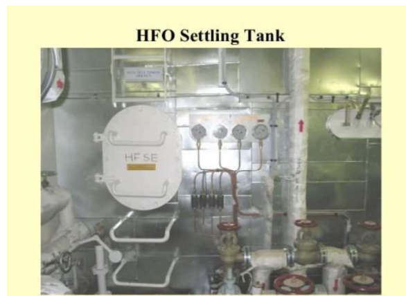
Gambar 2. 7 Settling Tank Sumber: (www.slideshare.net, 2019)
