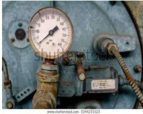
Gambar 2. 8 Pressure Gauge
