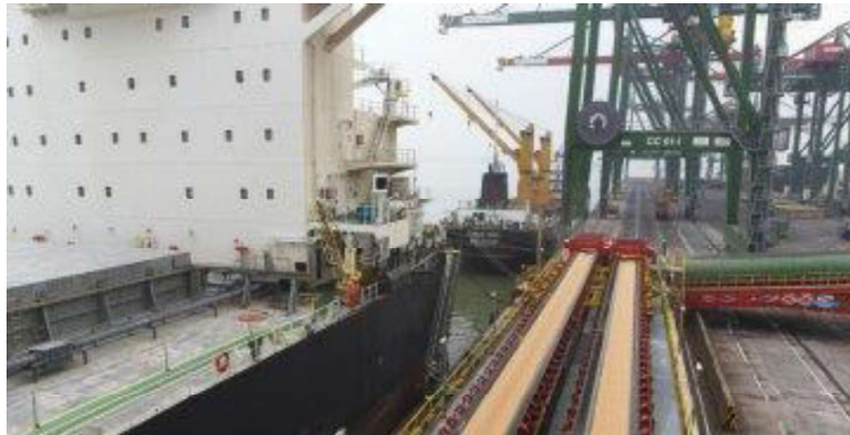
Gambar 2. 4 Conveyor PT. Terminal Teluk Lamong
