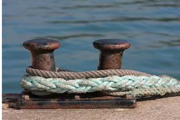
Gambar 2. 16 Mooring post Sumber: freeimages.com
