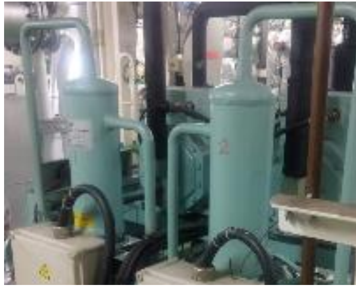
Gambar 2. 5 Oil Separator
