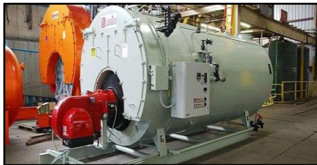
Gambar 2. 2 Boiler
